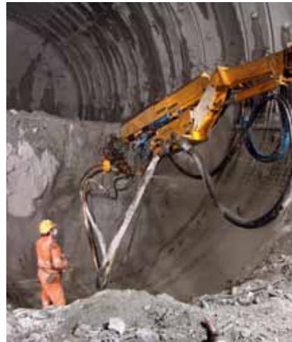
Fig. 3-9: Método de impulsar la corona [Driving of Crown method]
