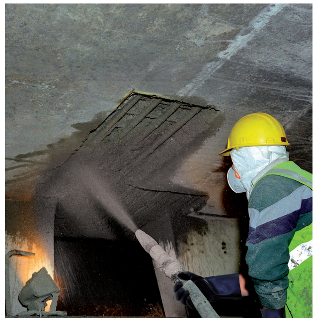
Sprayed mortar
