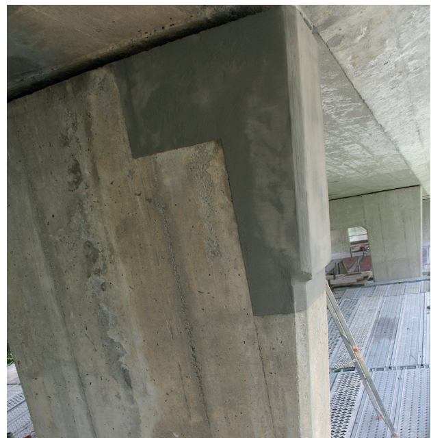
Repair work completed
