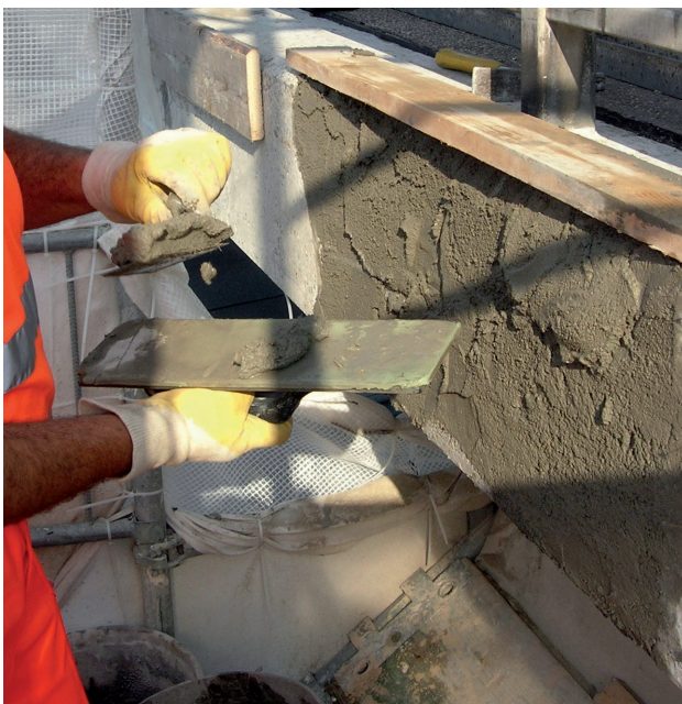
Hand applied mortar
